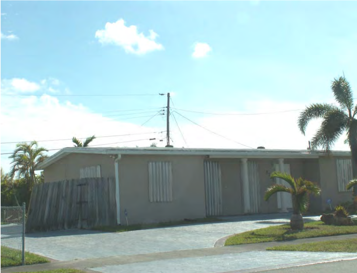
View of well prepared home which suffered no hurricane damage.
