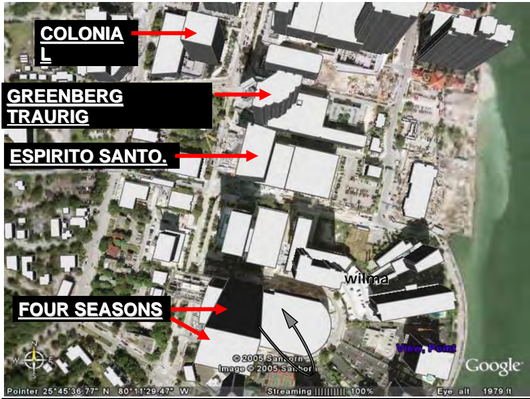
View of damaged buildings in the Brickell area.
