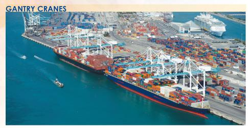
13 ship-to-shore cranes including six super Post-Panamax, the largest in the Southeastern U.S. The cranes have an outreach of 22 containers wide, stack up to nine containers high above deck, and 11 containers below deck with no height restrictions.
