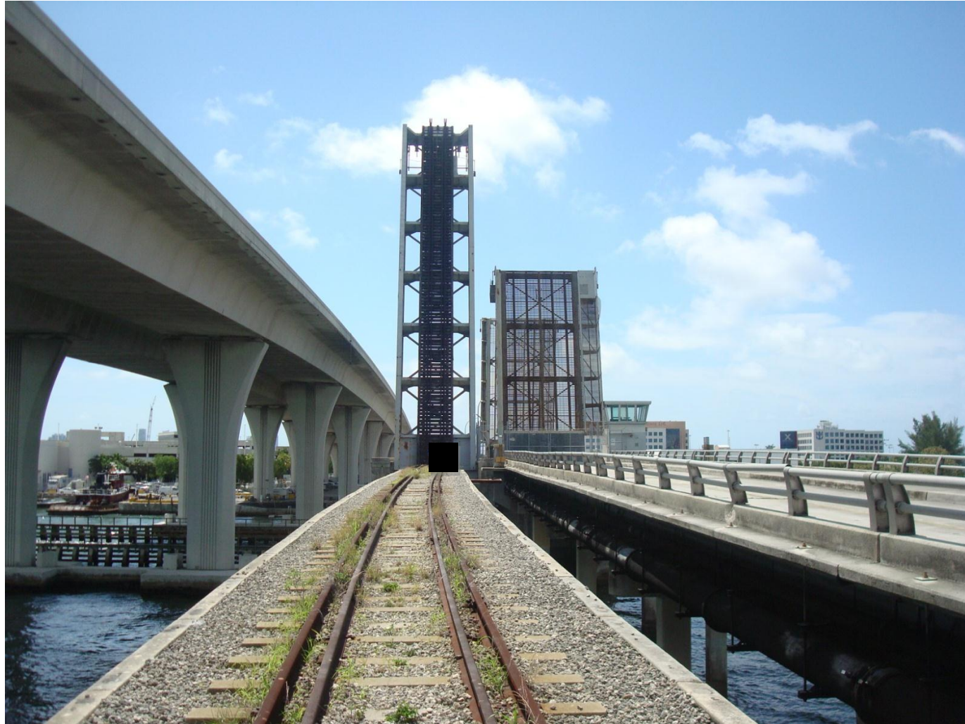
FIGURE 5.21: EXISTING ROADWAY AND BASCULE BRIDGE
